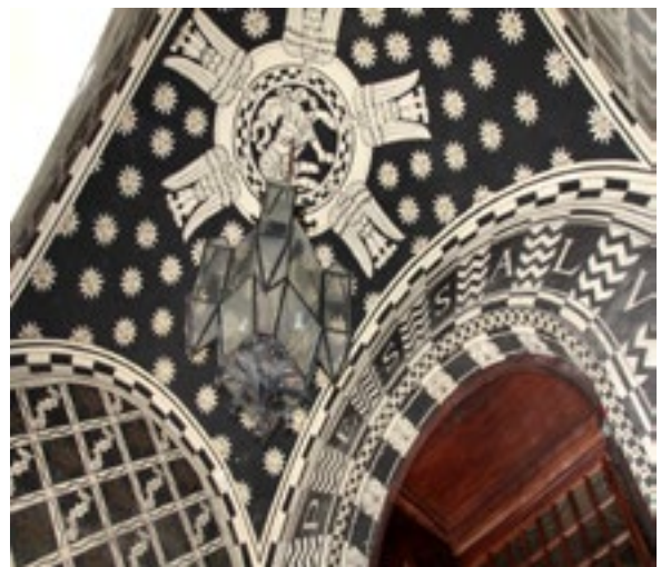
Front porch ceiling
